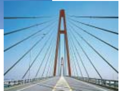
Bridge Guy Lines
